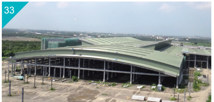
屏东县潮州台铁客车及机车维修厂屋顶 / 侧墙，PVDF 烤漆钢板 Roofing/Siding of Taiwan Railways Administration Chaozhou Coach Yard, Pingtung, Taiwan Paint Type: PVDF
