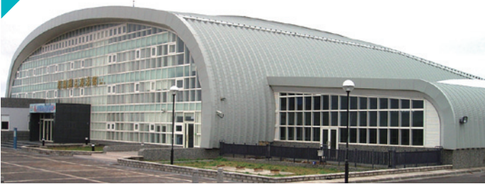
澎湖县立游泳馆屋顶 / 侧墙，PVDF 烤漆钢板 Roofing/Siding of Penghu County Swimming Pool, Penghu, Taiwan Paint Type: PVDF
