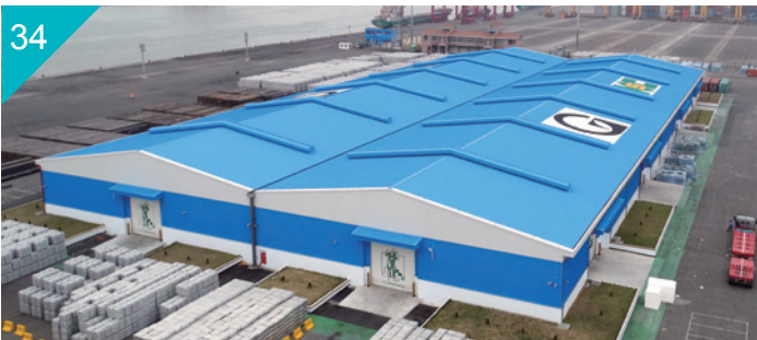
高雄港 122 号码头第三栋物流仓库屋顶 / 侧墙，PVDF 烤漆钢板 经销 / 士兴集团 Roofing/Siding of the 3rd logistics warehouse at Dock No. 122, Port of Kaohsiung, Taiwan Paint Type: PVDF
