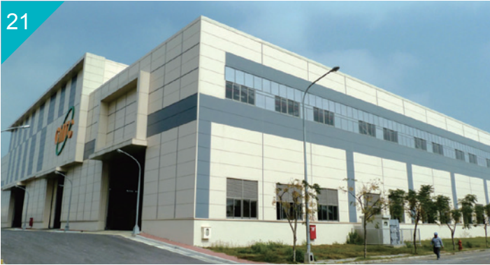
台南荣钢材料科技精炼厂屋顶 / 外墙，3C PVDF 洁冷烤漆钢板 Roofing/Siding of Gloria Material Technology Corp., Tainan, Taiwan Paint Type: PVDF Clean ColorCool
