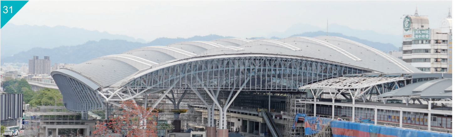
台湾铁路管理局台中车站屋顶，PVDF 烤漆钢板 Roofing of Taichung Train Station of Taiwan Railways Administration Paint Type: PVDF
