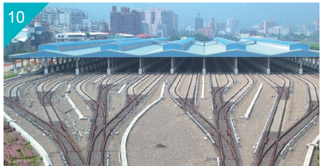
10 台北捷运土城机厂屋顶，PVDF 烤漆钢板 Roofing of Tucheng Depot of Taipei Rapid Transit Corp., Taiwan Paint Type: PVDF
