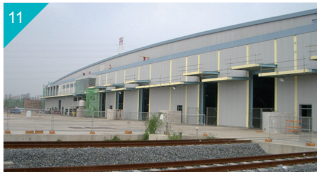
11 台湾高铁高雄燕巢总机厂屋顶 / 侧墙，PVDF 烤漆钢板 Roofing/Siding of Taiwan High Speed Rail–Yencho Main Workshop, Kaohsiung, Taiwan Paint Type: PVDF
