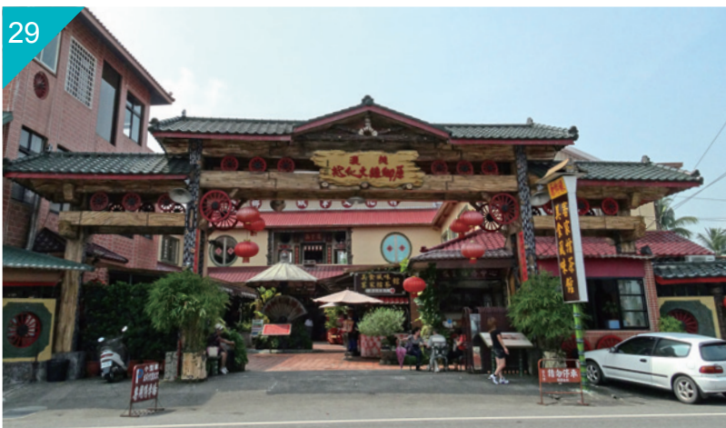
美浓原乡缘民俗村屋顶钢瓦 PVDF 烤漆钢板 Metal Tile of Meinung Folk Village, Kaohsiung, Taiwan Paint Type: PVDF
