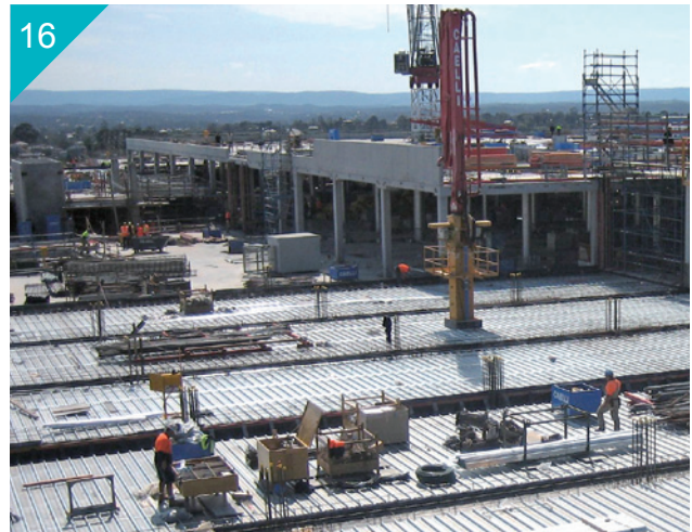
楼承板 ( 澳洲墨尔本皇家儿童医院实照 ) 热浸镀 5% 铝-锌钢板 Floor Decks of the Royal Children's Hospital in Melbourne, Australia Hot-Dip 5% Al-Zn Coated Steel Sheet
