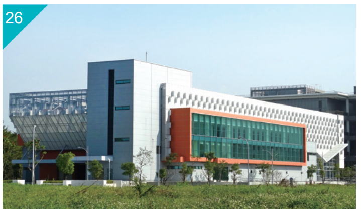
屏东农业生物科技园区侧墙，PVDF 钢板 Siding of Pingtung Agricultural Biotechnology Park, Taiwan Paint Type: PVDF
