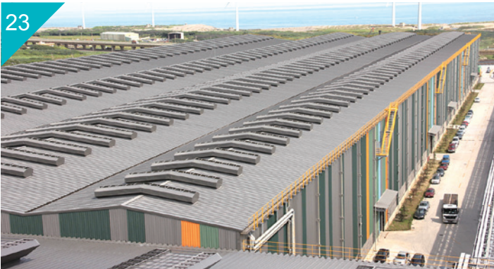
桃园县东和钢铁企业(股)公司屋顶 / 外墙，PVDF 烤漆钢板 Roofing/Siding of Tung Ho Steel Enterprise Corp., Taoyuan, Taiwan Paint Type: PVDF
