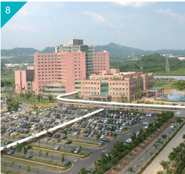
8 高雄市义大医院空中走廊屋顶 PVDF 烤漆钢板 Roofing of Sky Corridor, E-Da Hospital, Kaohsiung, Taiwan Paint Type: PVDF
