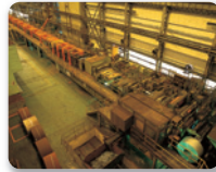
酸洗线 Push-Pull Pickling Line
