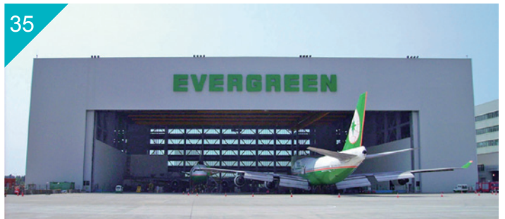
桃园长荣航太(股)公司第三飞机维修棚厂屋顶 / 侧墙，PVDF 烤漆钢板 Roofing/Siding of the 3rd Hangar of Evergreen Aviation Technologies Corp., Taoyuan, Taiwan Paint Type: PVDF
