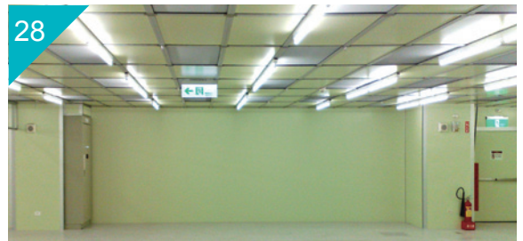
日月光中坜厂房抗静电无尘室, 抗静电烤漆钢板 Clean Room of Advanced Semiconductor Engineering Inc., Jungli, Taiwan Anti-Electrostatic Polyester Pre-Painted Steel Sheet
