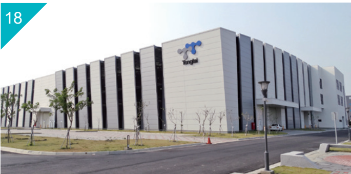
高雄科学园区东台精机(股)公司室外三明治板 洁净节能(3C)高耐磨耗(RA)及高耐磨耗(RA) PVDF 烤漆钢板 Sandwich Panels for Outdoor Use at Tongtai Machine & Tool Co., Ltd., Kaohsiung Science Park, Taiwan Paint Type: RA PVDF & 3C-RA PVDF
