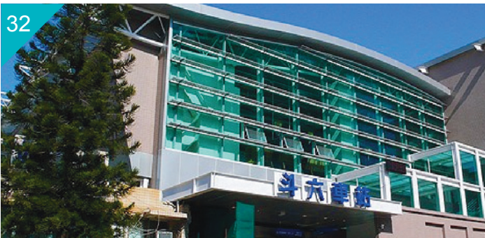
台湾铁路管理局斗六车站屋顶 / 侧墙，PVDF 烤漆钢板 Roofing/Siding of Douliou Station of Taiwan Railways Administration, Yunlin, Taiwan Paint Type: PVDF
