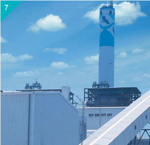
7 云林县台塑石化工业轻油裂解厂厂房 高膜厚 PVDF 烤漆钢板 Naphtha Cracking Plant, Formosa Petrochemical Corporation, Yunlin, Taiwan High Build PVDF Pre-Painted Steel Sheet
