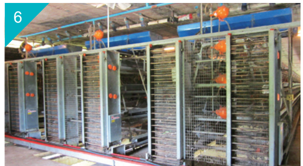
鸡舍结构支架 (泰国)，热浸镀 5% 铝-锌钢板 Frame of a Hen House (Thailand) Hot-Dip 5% Al-Zn Coated Steel Sheet
